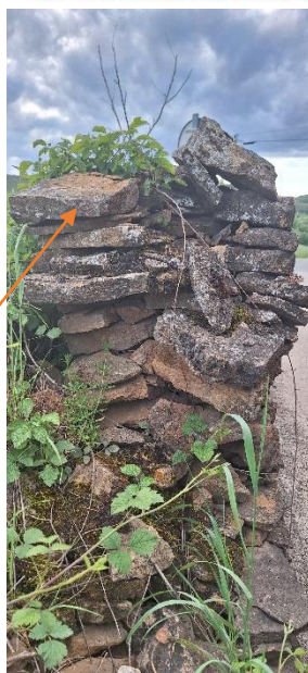
Cross section through the middle of the dry stone wall
